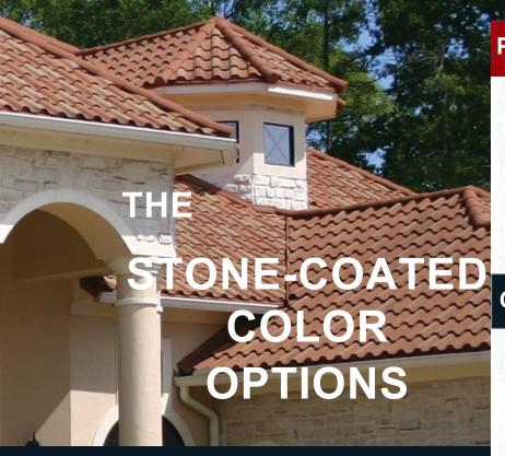
THE STONE-COATED COMES IN THE FOLLOWING PROFILES AND COLOR SELECTIONS. EACH COLOR IS A MIXTURE OF THREE GRANULE COLORS EMBEDDED IN ADHESIVE ON 26 GAUGE GALVALUME STEEL.
